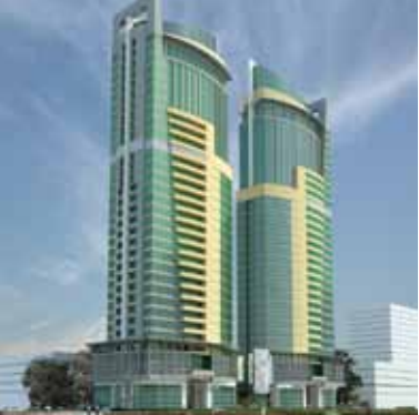
PSPF Commercial Towers
